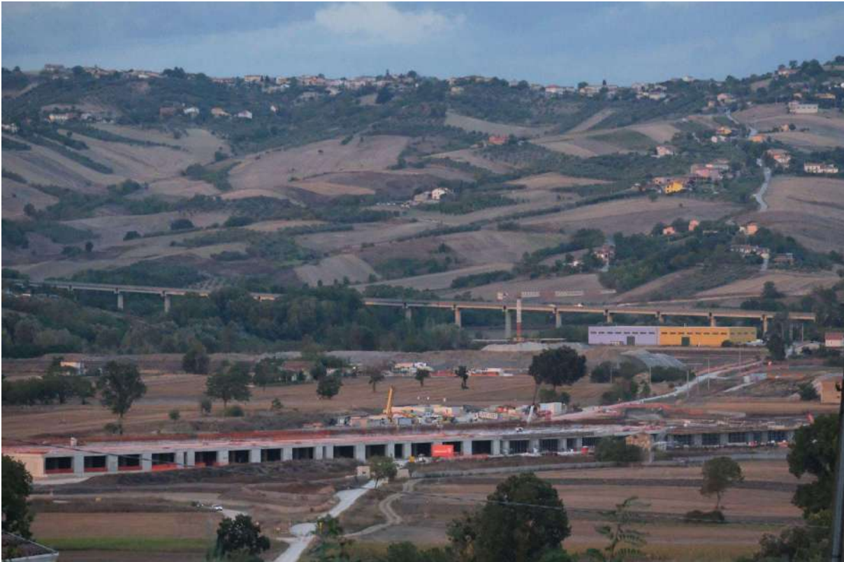
Figure 17: HS/HC station and railway building site.
